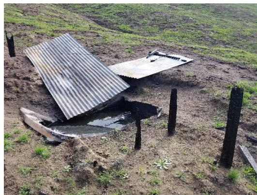
(Burnt Guzzler Scheduled for Repair)
