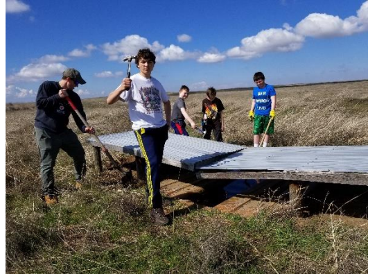
(Boy Scouts Repairing Guzzler)
